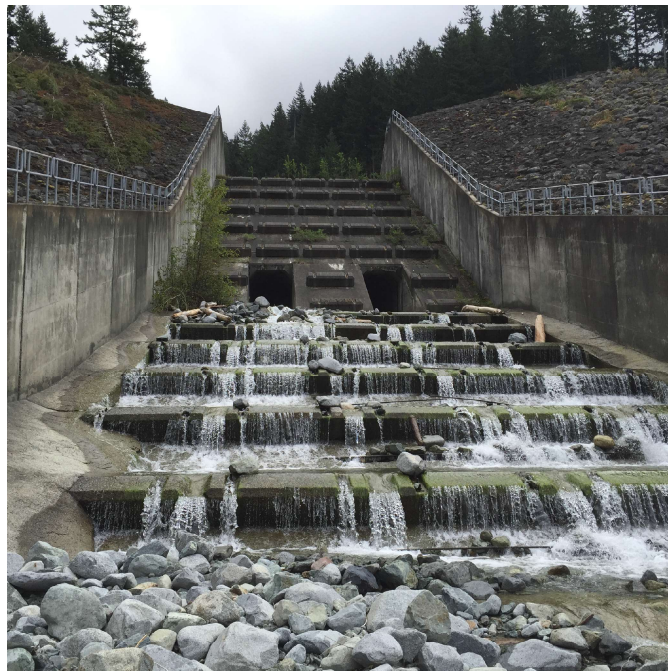
Recent activity on the debris flow retention structure, Sea to Sky highway, Lions Bay, BC. Photo by Michele Koppes
